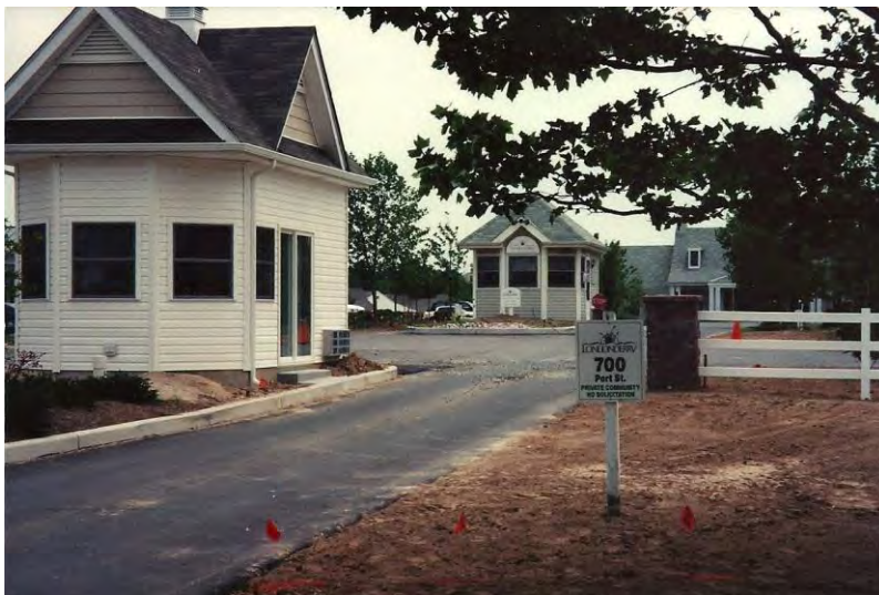
New Guardhouse Nearing Completion
