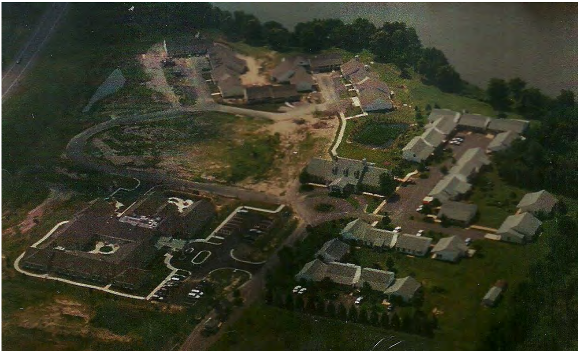
HeartFields and Phase II Cottages Under Construction
