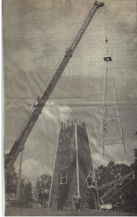
Restoration Under Way
