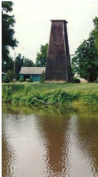
Windmill Before Restoration
